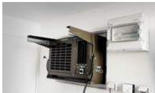
Container installation - inside view
