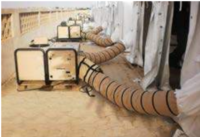
Installation with the air ducts
