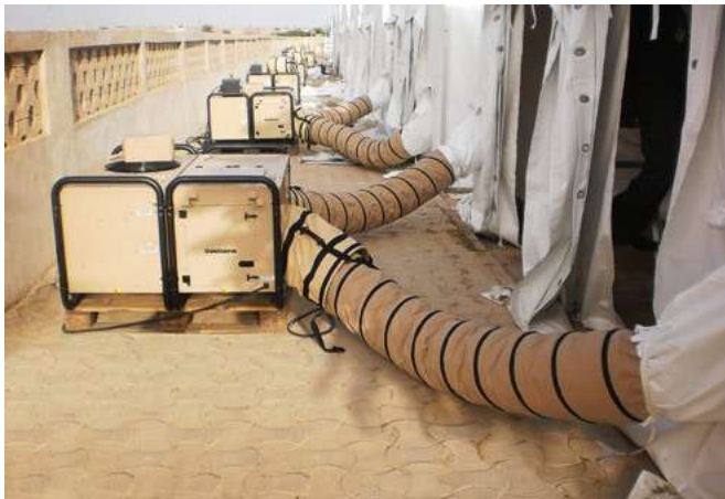
Installation with the air ducts
