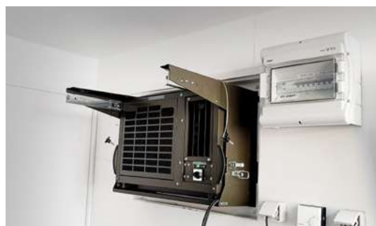
Container installation - inside view
