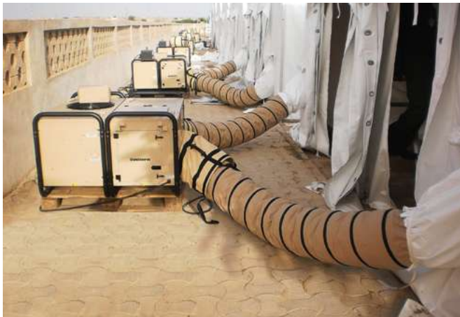
Installation with the air ducts
